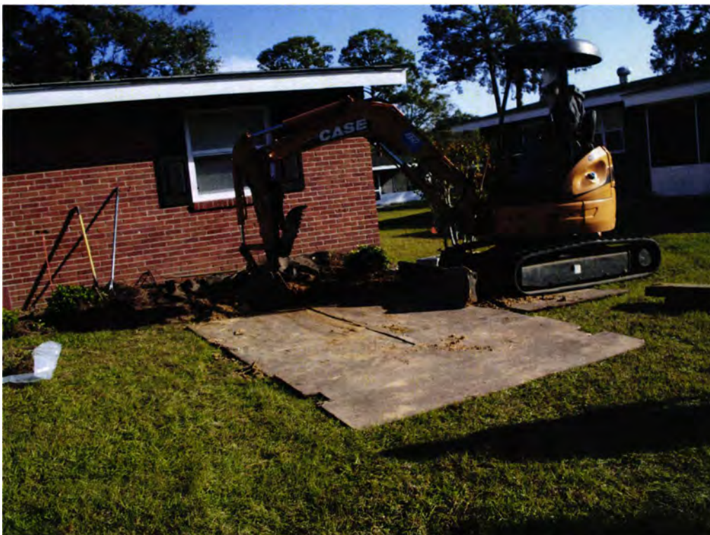
Picture 2: UST 515LaurelBB excavation in progress.
